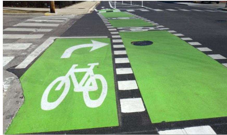
Figure F-24: Intersection Crossing Marking
