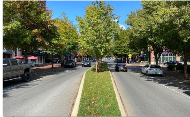
Figure F-19: Concrete Island
