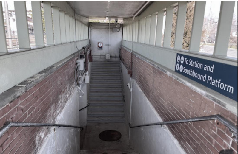
Figure 6-10: Aberdeen Amtrak/MARC Station
