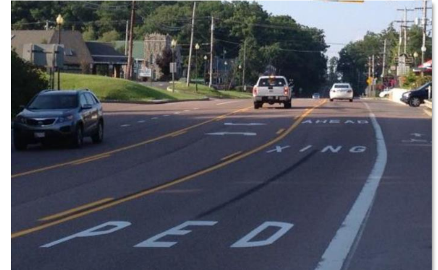
Figure F-20: In Pavement Text Markings
